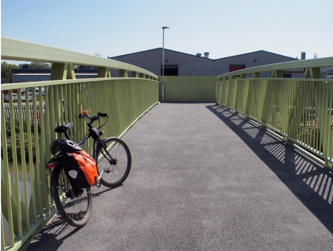
Figure 5 – Newly constructed 3.5m shared use bridge in Woodloes, Warwick
