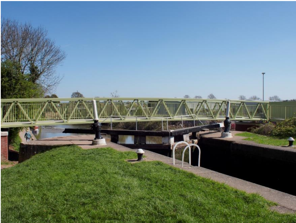
Figure 4 – Newly constructed shared use canal bridge in Woodloes, Warwick
