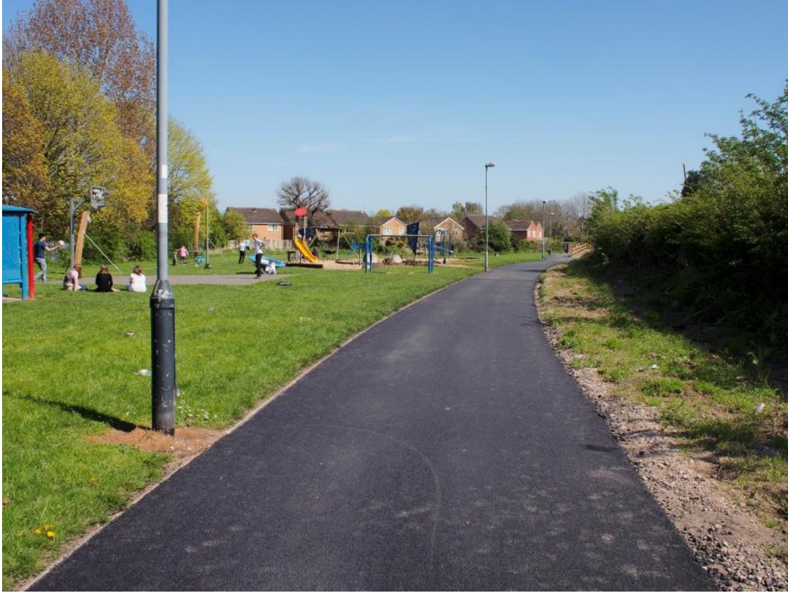
Figure 3 – Newly constructed shared use route in Woodloes, Warwick
