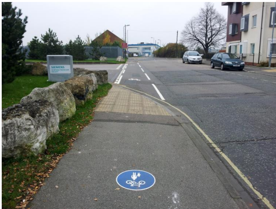
Figure 4 – Thermoplastic shared use symbol in Southampton
