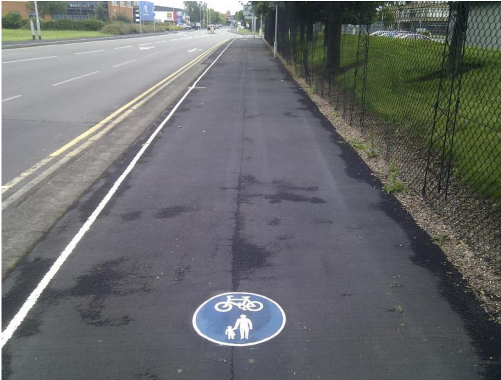
Figure 6 – Thermoplastic shared use symbol in Loughborough
