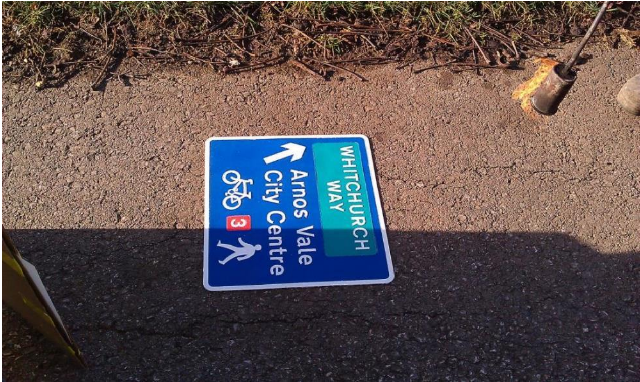
Figure 3 – Thermoplastic route signing
