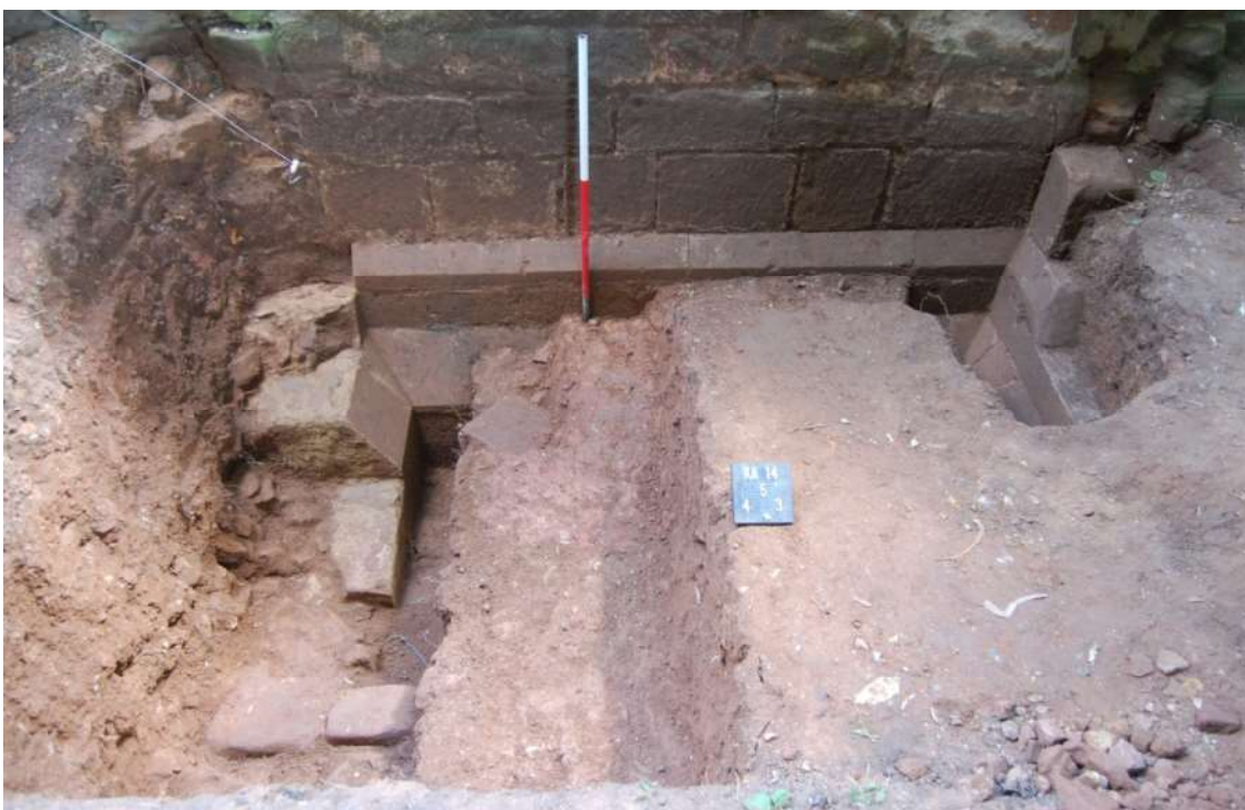
Fig 4: The remains of both probable buttresses and the lower part of the gatehouse wall
