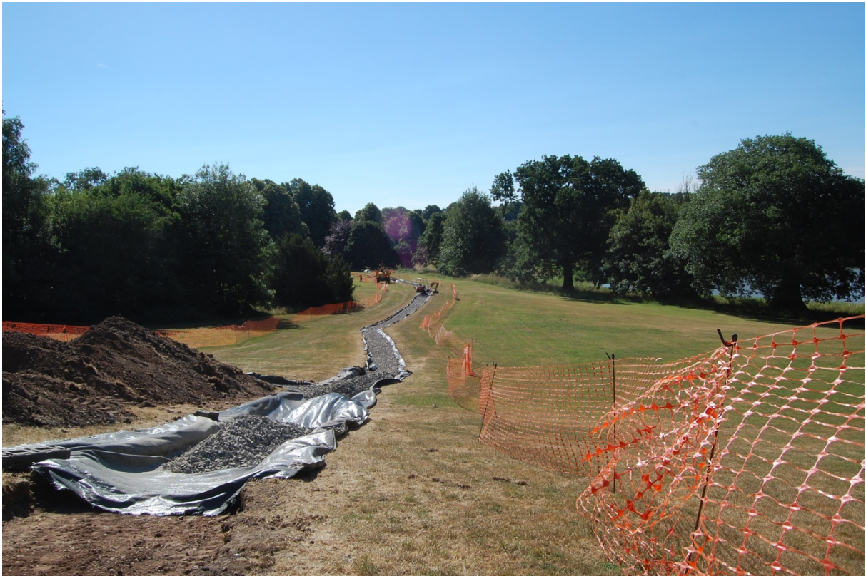
5: Geotextile permeable membrane and base course being positioned following trench excavation and recording of archaeological features. View south-east from top of hill at the site's western end
