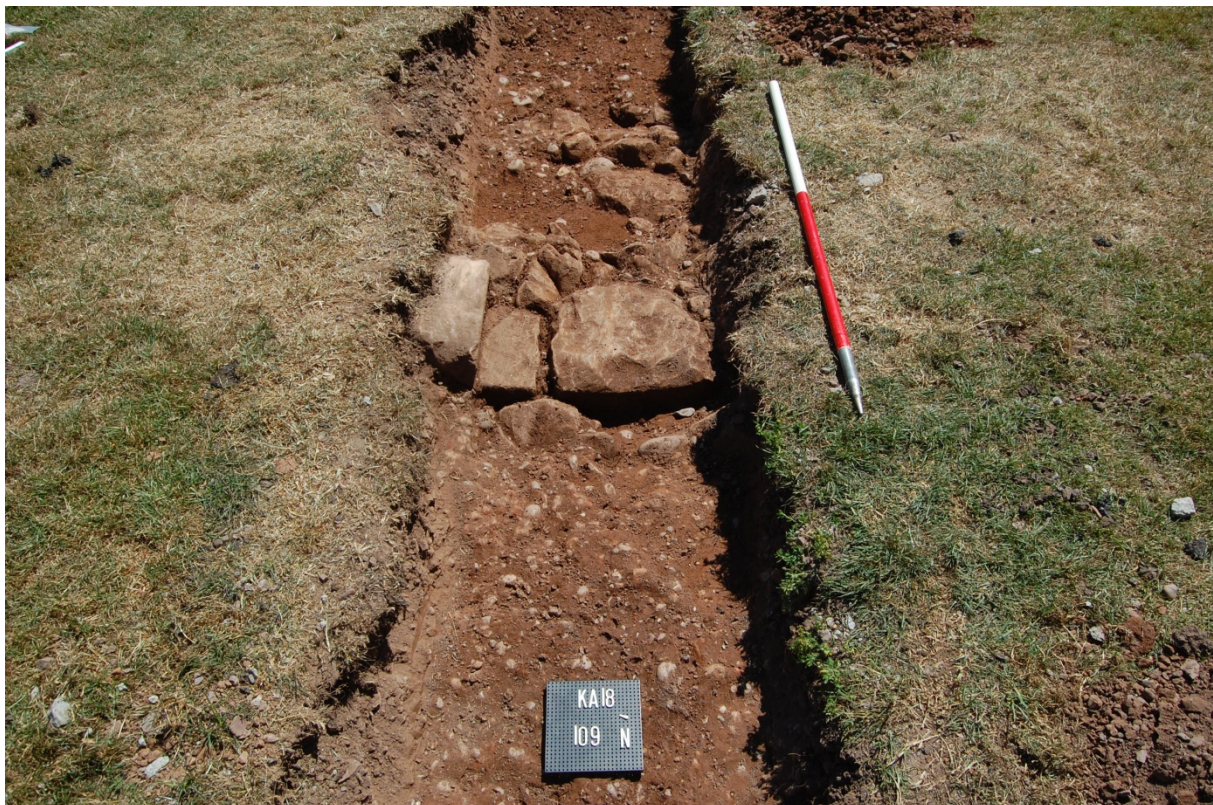
8: Wall 109, looking north-west following its initial discovery and prior to trench widening with a toothless bucket
