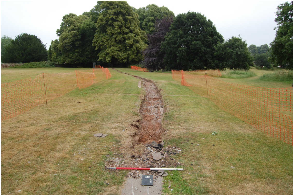
1: Removal of modern tarmac path 100 in progress, looking east
