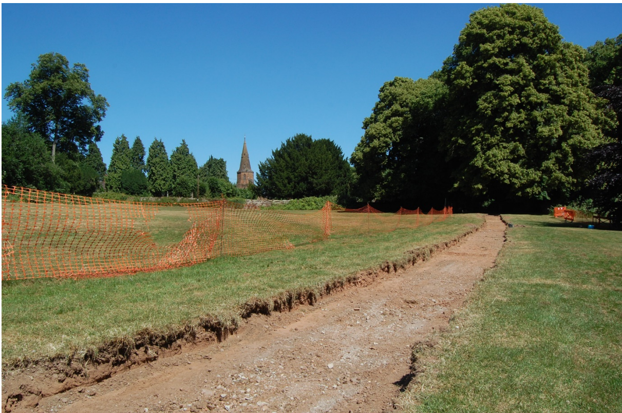
4: The new footpath trench with St Nicholas Church beyond, looking north-east
