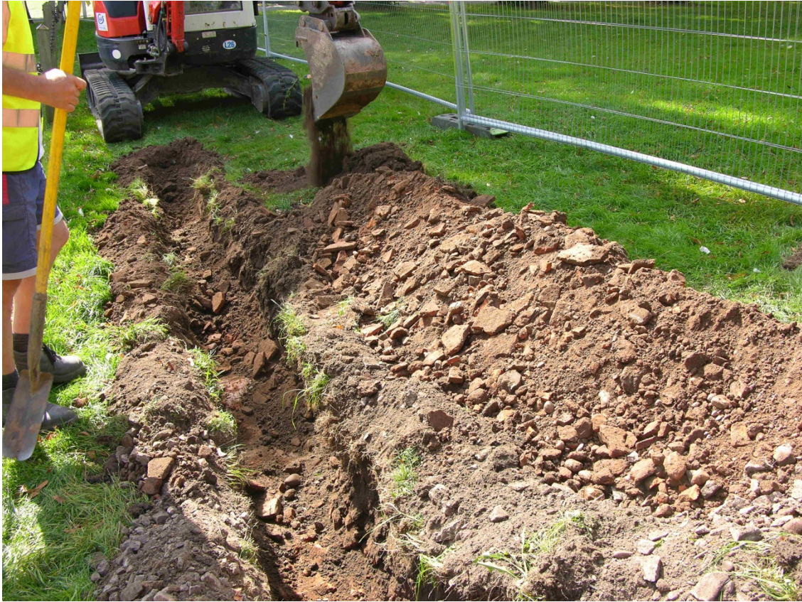
Fig. 3: Excavating through demolition layer 9, on west side of car park
